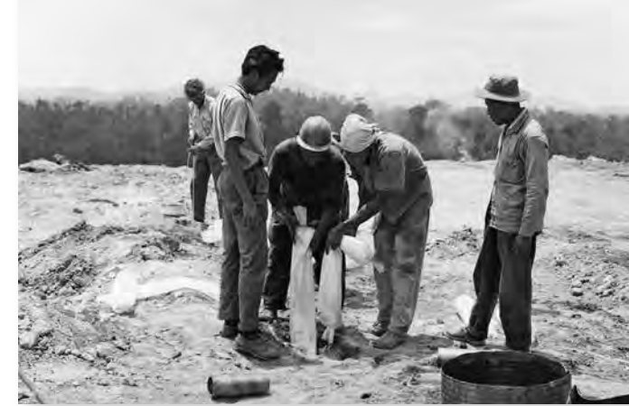
Fertilizer was the main explosive in blast holes.
