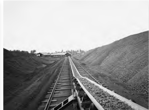
(from left) At the Sura terminus, ore wagons were dumped. Then the ore went seaward to ships or landward into stockpiles.
