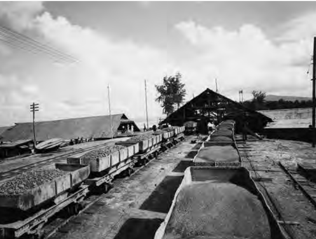
(from left) At the Sura terminus, ore wagons were dumped. Then the ore went seaward to ships or landward into stockpiles.
