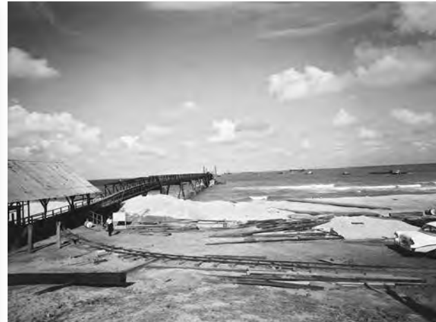
(from left) At the Sura terminus, ore wagons were dumped. Then the ore went seaward to ships or landward into stockpiles.
